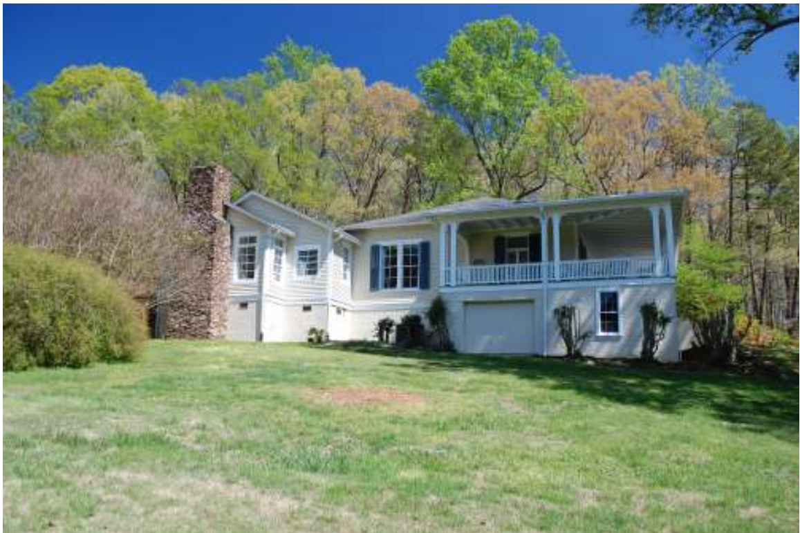
Gen. Robert F. Hoke Cottage, West Elevation
