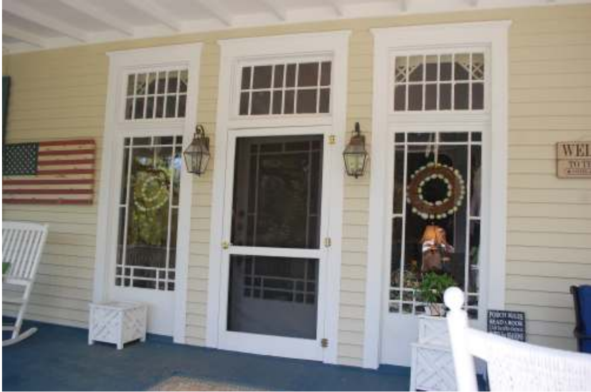
Gen. Robert F. Hoke Cottage, South Elevation, Front Entry
