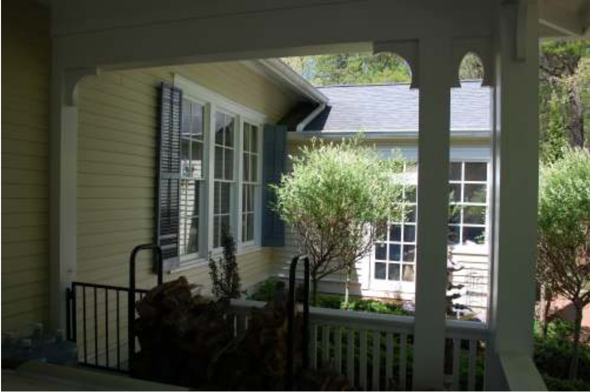
Gen. Robert F. Hoke Cottage, East Elevation, 1997 addition (View from porch)
