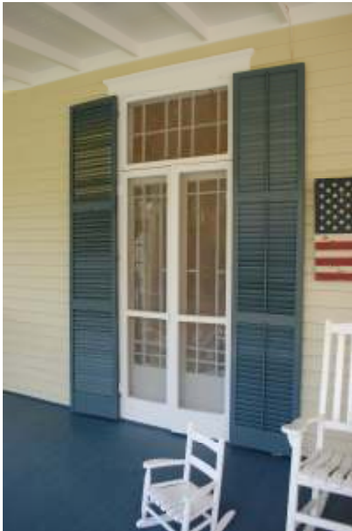
Gen. Robert F. Hoke Cottage, South Elevation, Front Porch
