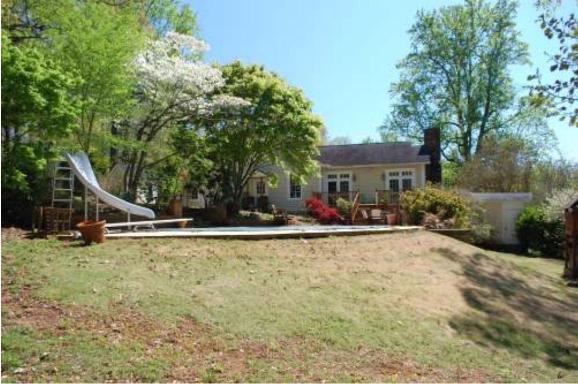
Gen. Robert F. Hoke Cottage, North elevation
