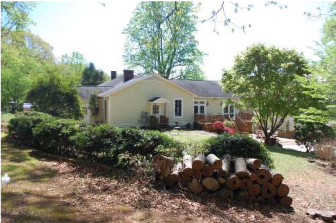
Gen. Robert F. Hoke Cottage, North elevation
