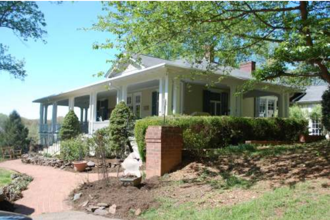
Gen. Robert F. Hoke Cottage, Southeast corner
