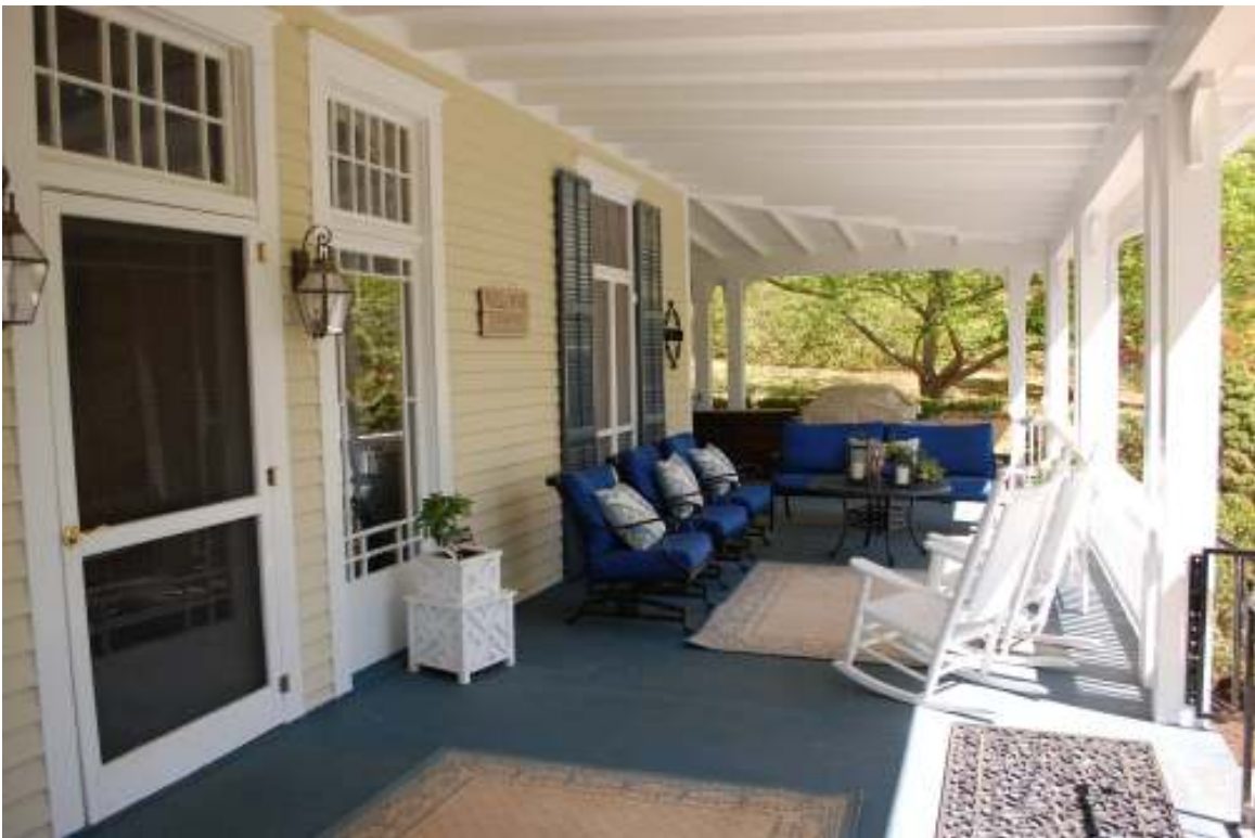
Gen. Robert F. Hoke Cottage, South Elevation, Front Porch
